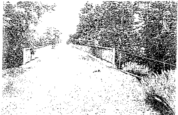
4 - Bridge over Vineyard Ave
